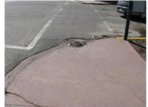
Photo 15 Catchbasin in Middle of Crosswalk
