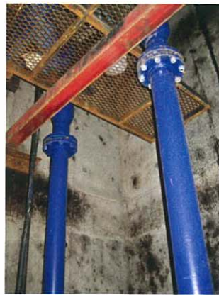
Discharge piping and support beam
