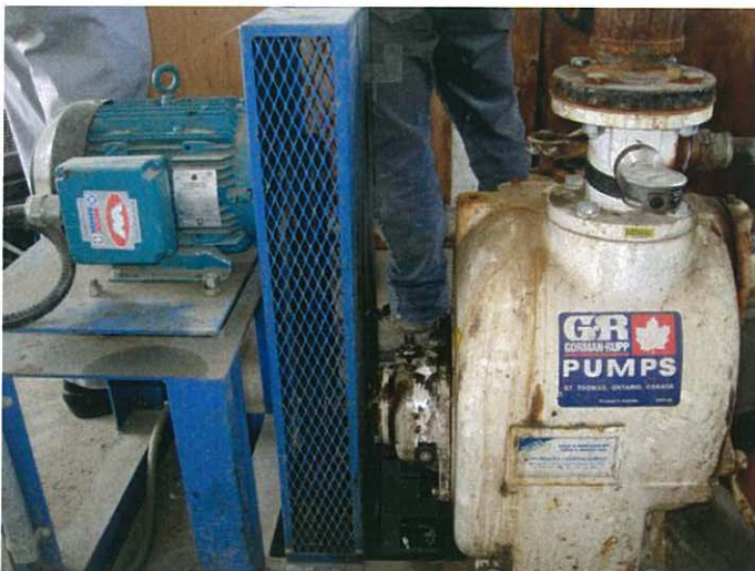
Self-priming sewage pump; wet well
