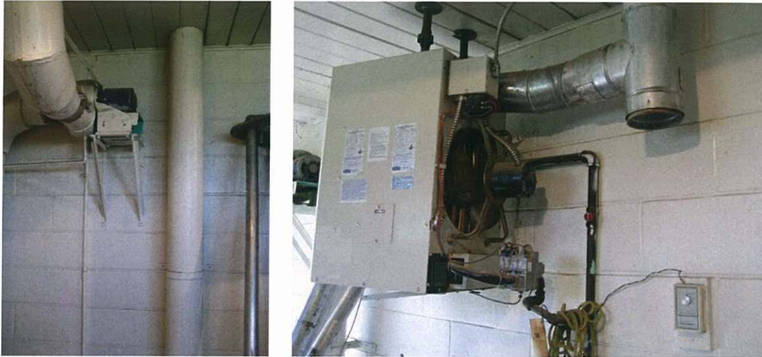
Ventilation system; gas heater
