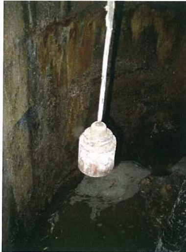
Ultrasonic level sensor
