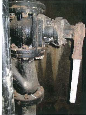
Discharge isolation valve
