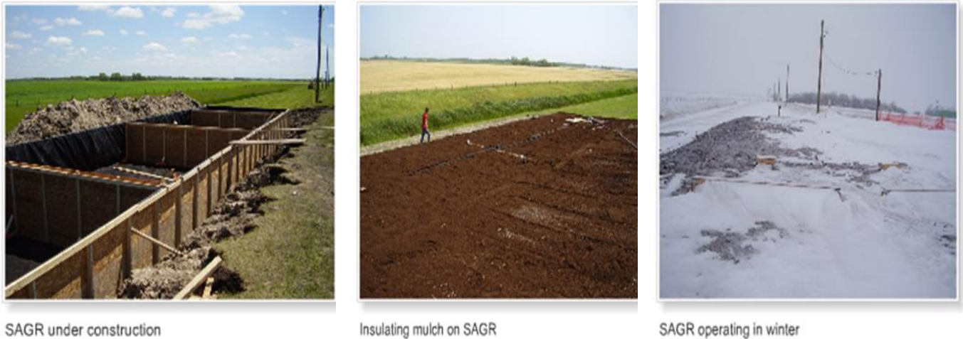
Figure 6-8 SAGR System Installation during Construction, and Summer and Winter after Construction
