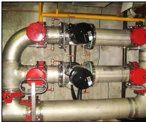
Figure 3-3 Existing UV Disinfection
