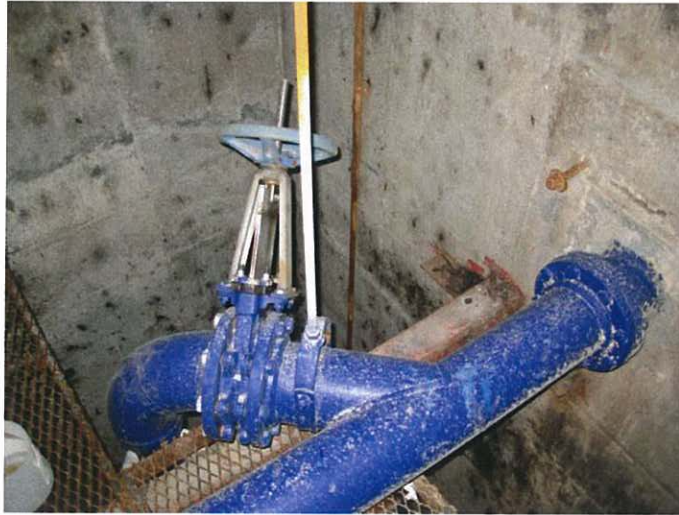
Discharge isolation valve
