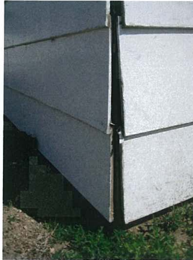
Damaged siding
