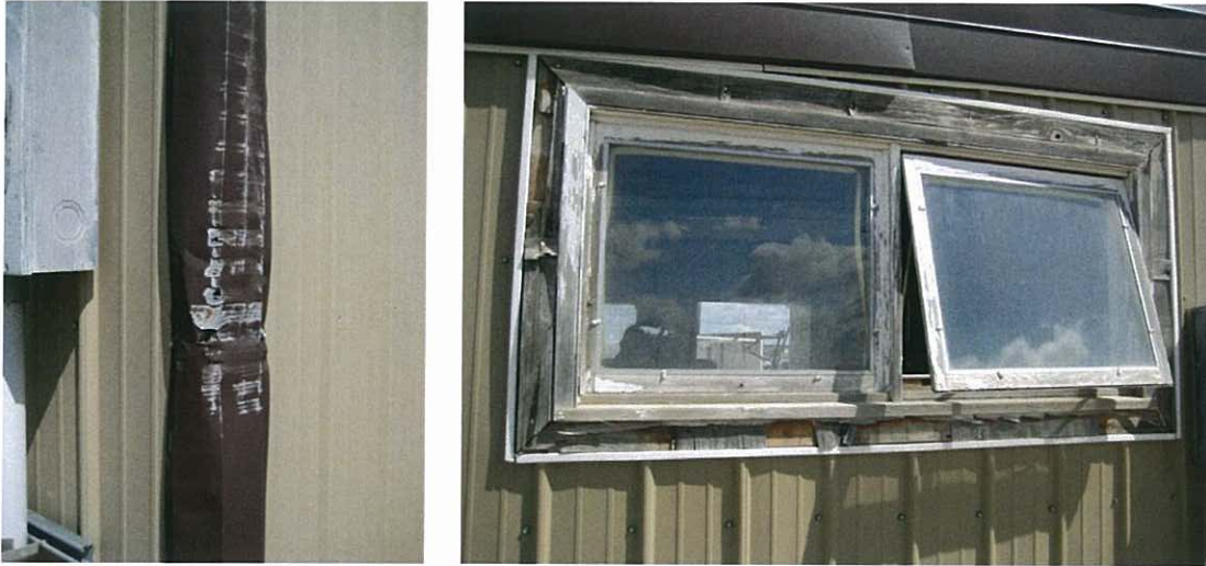
Damaged siding and window
